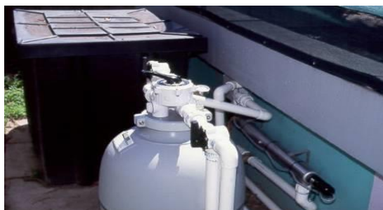
Three types of filtration- Mechanical (Grey pond filter), Biological (black tub with dense matting) and UV Clarification/Sterilisation (Stainless steel tube)
